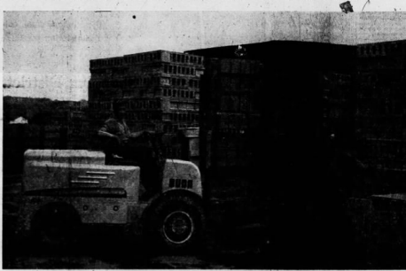
The latest type BLOCK LIFTER shown here, is used for placing cures in storage for curing. Steve Thompson is at the wheel. On the right is William S. Shaffer, owner and operator of the SHAFFER BLOCK WORKS.
